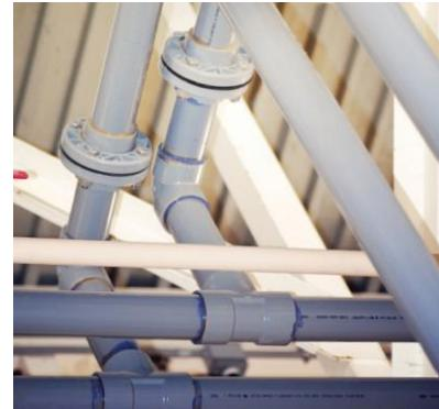
Corzan® Material and Piping Solutions offer a complete tie-in to tap solution made up of Schedule 80 pipe & fittings, flanges, valves, and specialty adapter fittings including: MIP Threads x CPVC, FIP Threads x CPVC, Stub Out Elbows, and Male Sweat Adapters. Potable water systems designed with Corzan CPVC offer the best solution for reducing biofilm buildup and the growth of Legionella while being immune to degradation caused by standard disinfection procedures.
