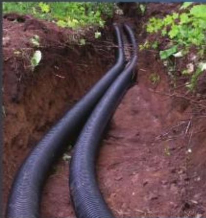
Ecoflex® pre-insulated piping
