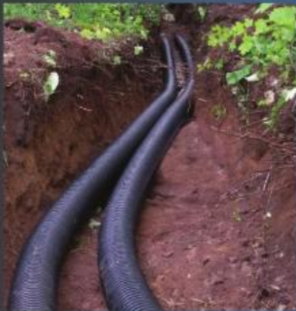
Ecoflex® pre-insulated piping
