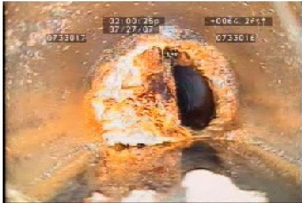
The main sewer line where the service connection from Bar an eating and drinking establishment connects.
